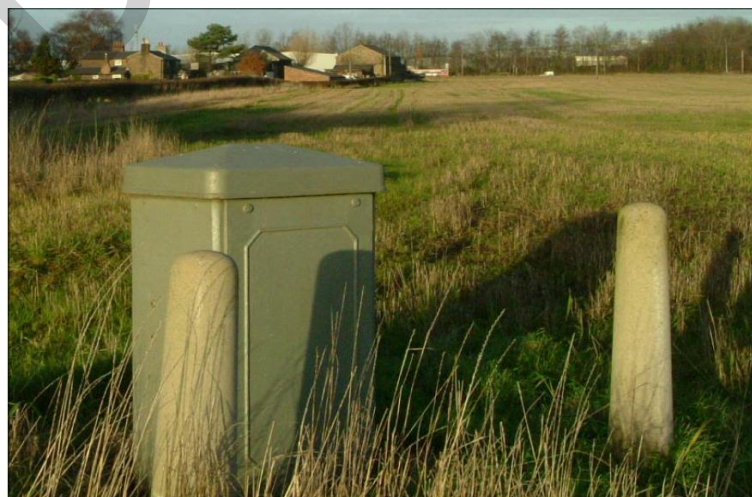
Figure 4.10: Photograph of Above Ground Inspection Kiosks for UGC
