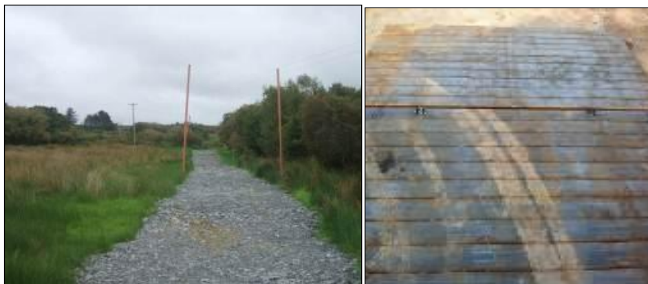
Figure 7.4: Temporary Stone Road and Wooden Sleepers
