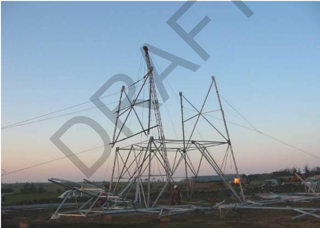
Figure 7.7: Derrick Pole at Tower Base
