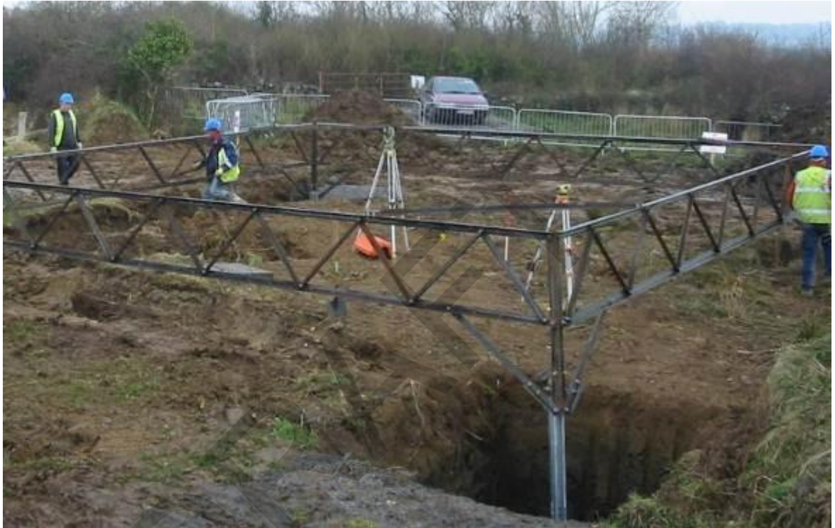
Figure 7.6: Photograph of Setting Template being prepared for Final Concreting
