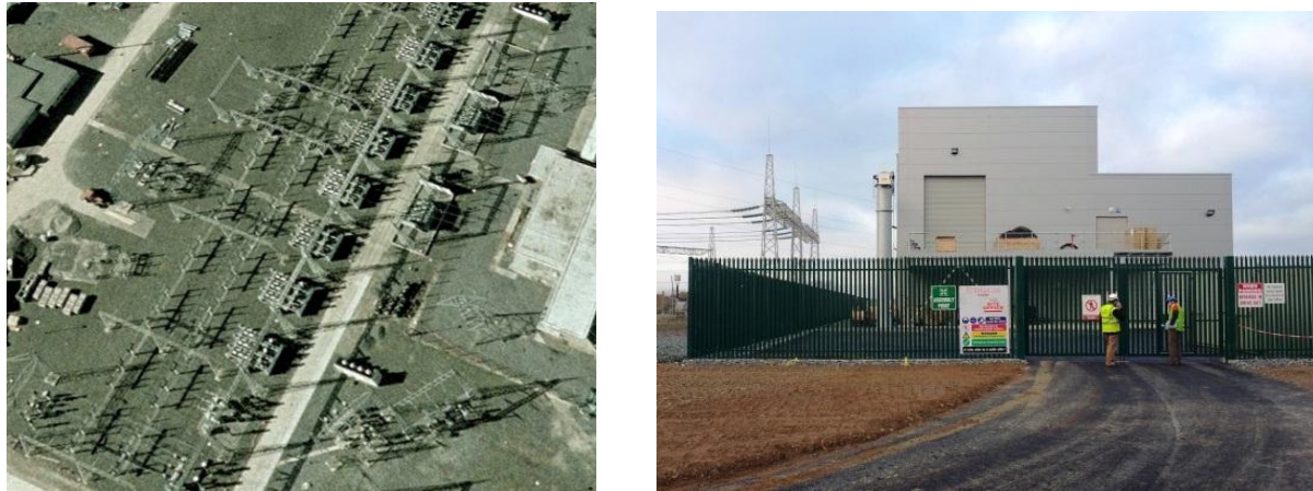
Figure 10.4: Typical AIS and GIS Substations
