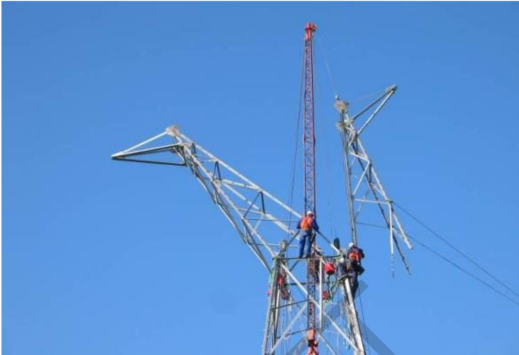
Figure 7.8: Lower Part of the Tower Head being dropped into Position
