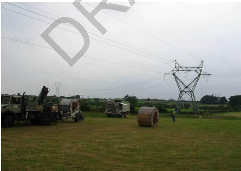
Figure 7.14: Typical Stringing Equipment
