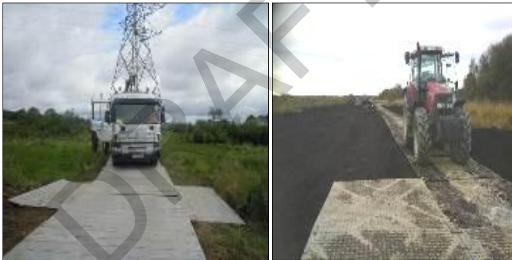
Figure 7.3: Temporary Aluminium and Rubber Panel Tracks
