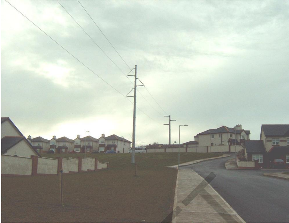
Figure 4.14: 110 kV Monopole Overhead Line in Cork
