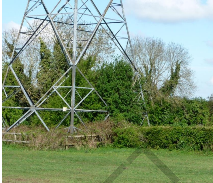
Figure 4.9: Photograph of a Tower Straddling a Hedgerow with Vegetation Re-established
